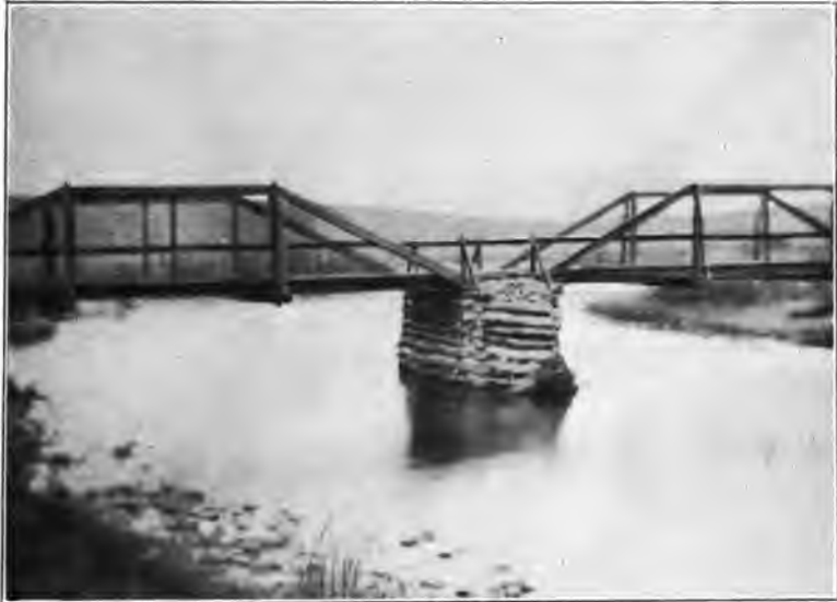
COUNTY HIGHWAY BRIDGE OVER STRAWBERRY RIVER NEAR THEODORE, WASATCH COUNTY.
